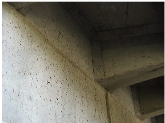
Figure 4. Heavy fecal accumulation from night-roosting
