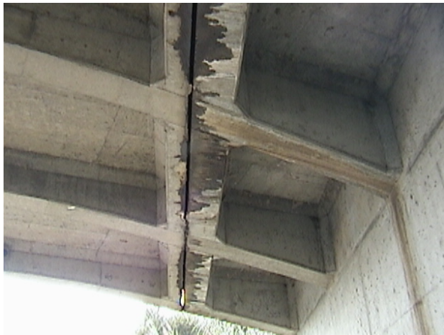
Figure 9. Heavy urine staining at expansion joints
