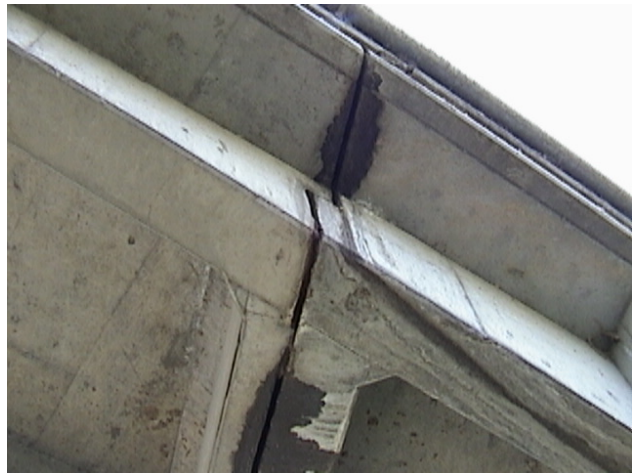
Figure 8. Expansion joint showing efflorescence/staining
