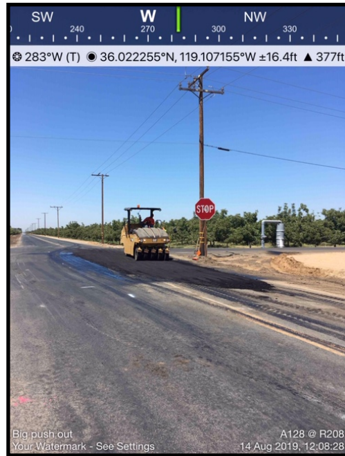
Replaced with new asphalt
