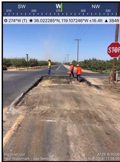
Removed distorted asphalt
