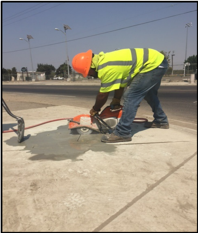
Cut sidewalk for sign installation in Poplar:
