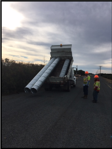
Continued culvert pipe and drain inlet maintenance
