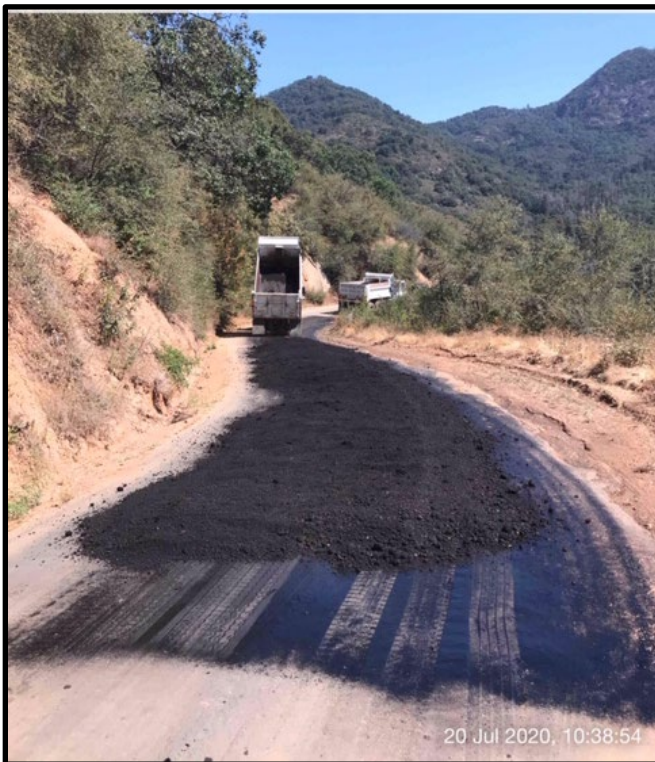
Blade patching on Mountain Road 276 near Mile Post 3.5
