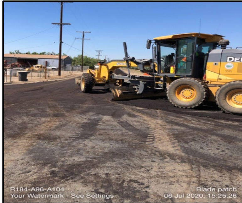
Blade patching on Road 184 between Avenue 96 and Avenue 104
