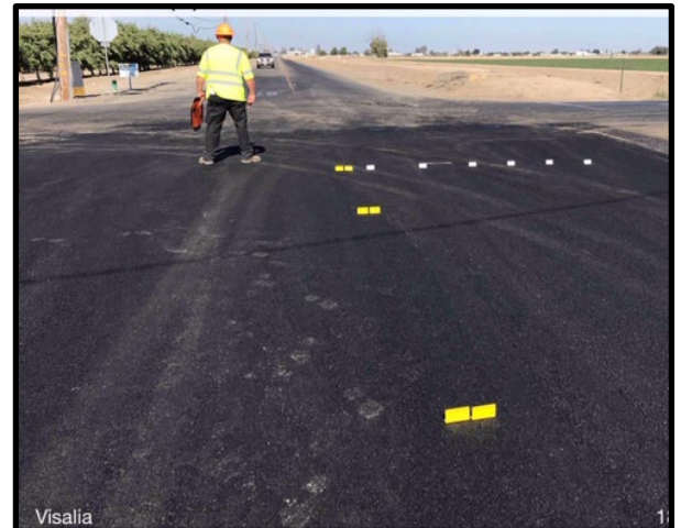
Grind and Overlay on Santa Fe, north of Avenue 272
