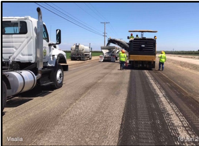
Grind and Overlay on Santa Fe, north of Avenue 272
