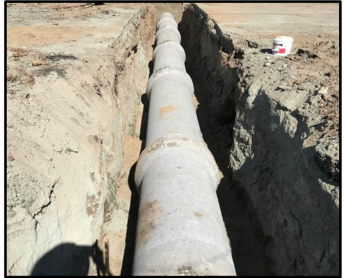
Road 234 storm drain pipe replacement
