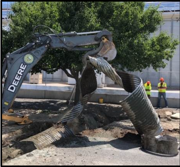
Road 234 storm drain pipe replacement
