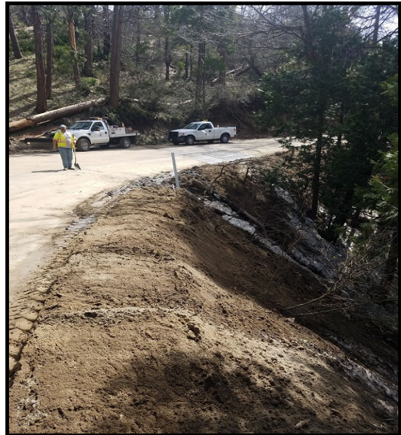
Repaired 5 locations for washouts
