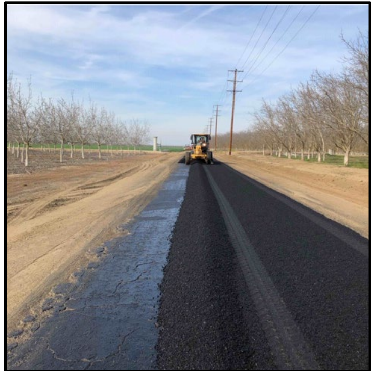
Blade patch at Road 176 between Avenue 128 and 136
