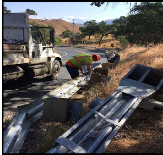
Repaired damaged guardrails on M137 (Reservation Road):
