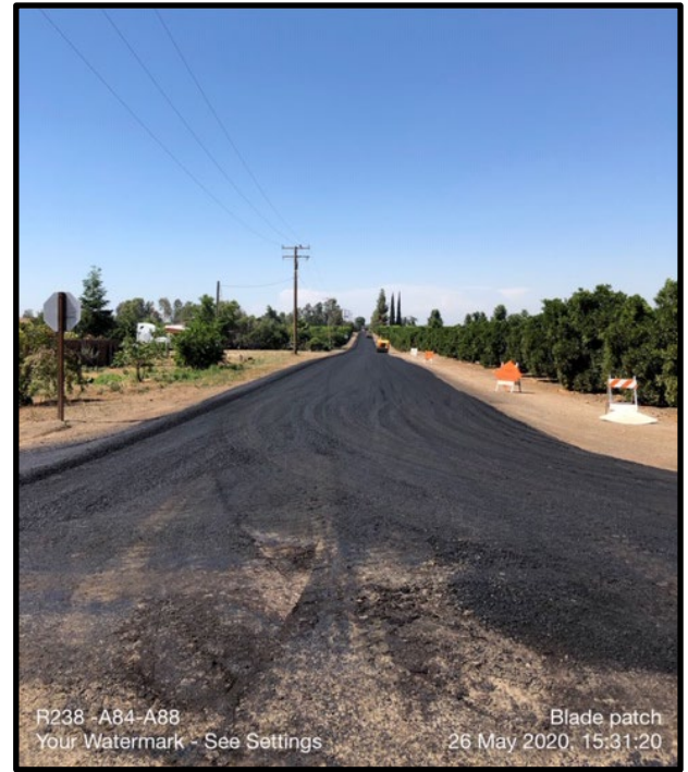
Blade patched Road 238 between Avenue 84 and Avenue 88
