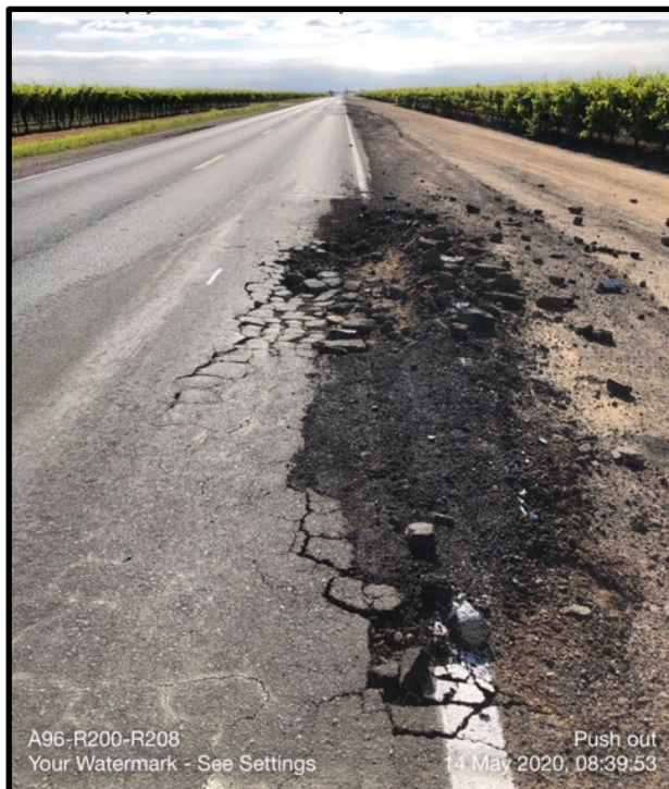
Repaired pavement edge failure on Avenue 96
