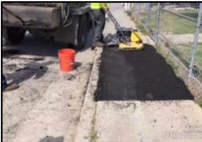
Temporary Sidewalk Repair in Pixley
