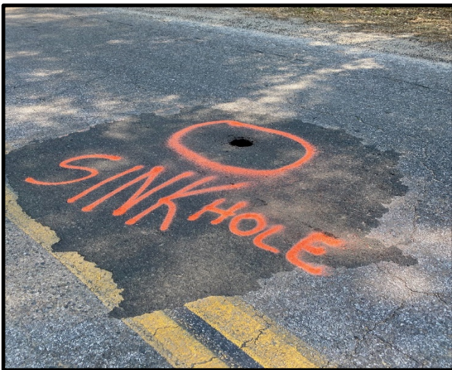
Repaired sinkholes on North Fork Drive
