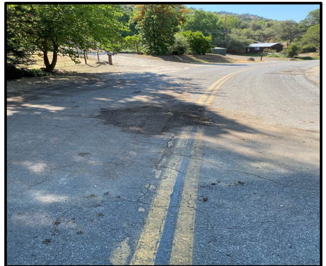
Repaired sinkholes on North Fork Drive
