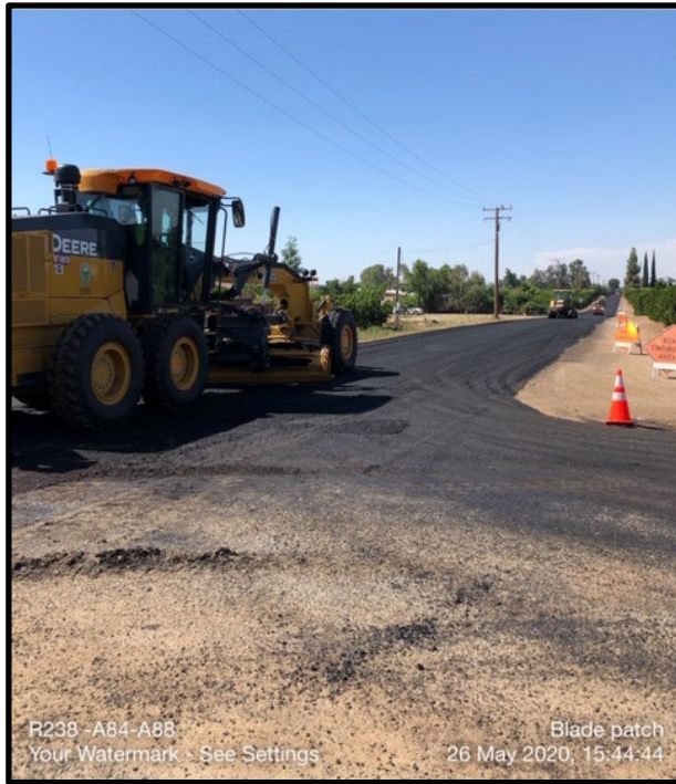
Blade patched Road 238 between Avenue 84 and Avenue 88
