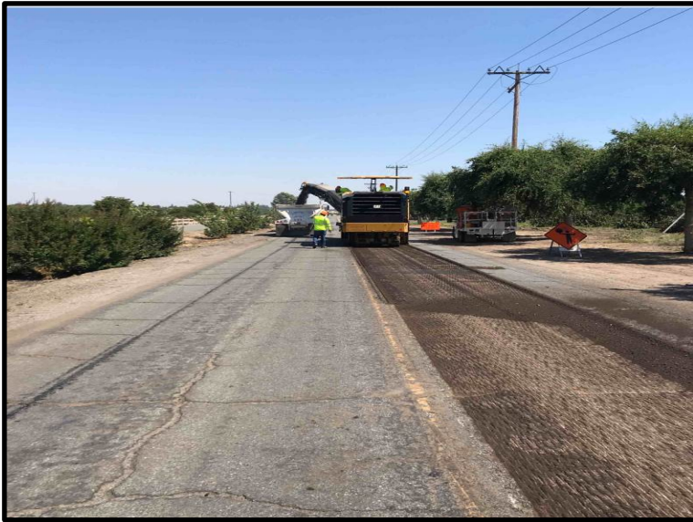
Pavement Grinding on Santa Fe at Avenue 272
