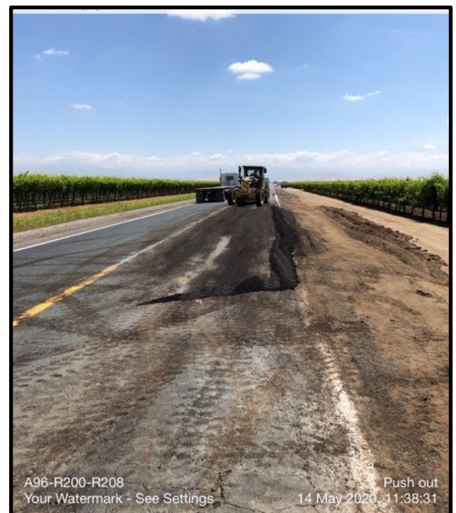
Repaired pavement edge failure on Avenue 96
