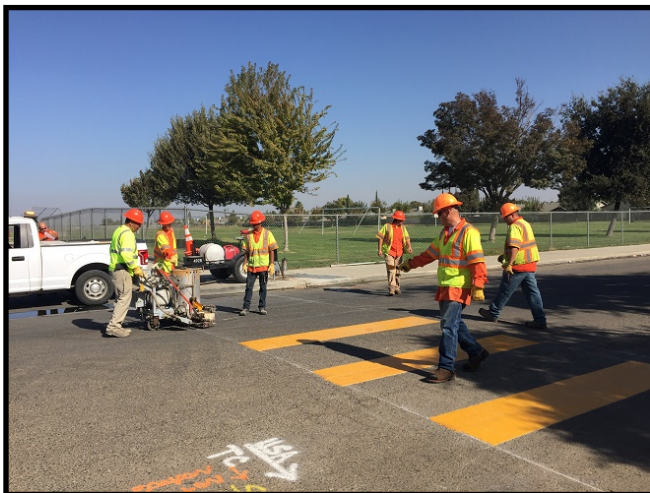
Installing ladder crosswalk
