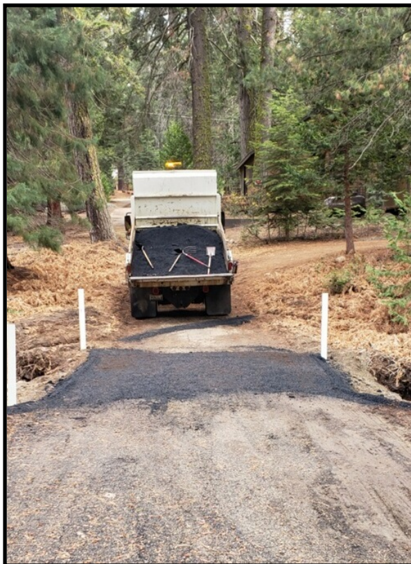
Picture 1- Asphalt patching over culvert pipe
