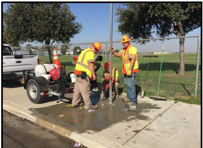
Drilling hole into concrete sidewalk to install post and sign
