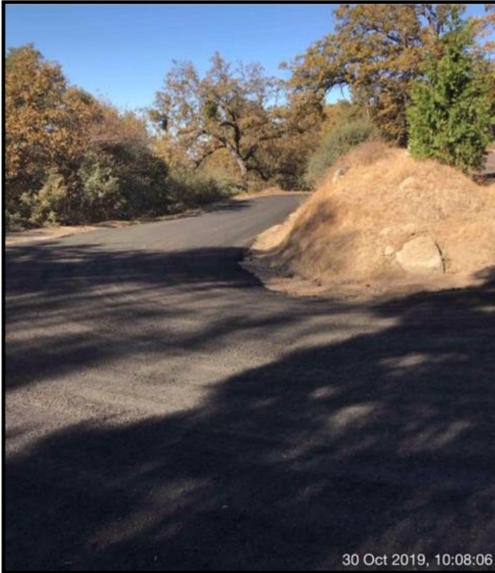
Blade patch on M296 near Springville (from MP 31 to 36)
