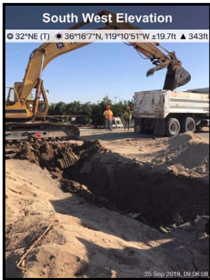
Removing old rusted pipe
