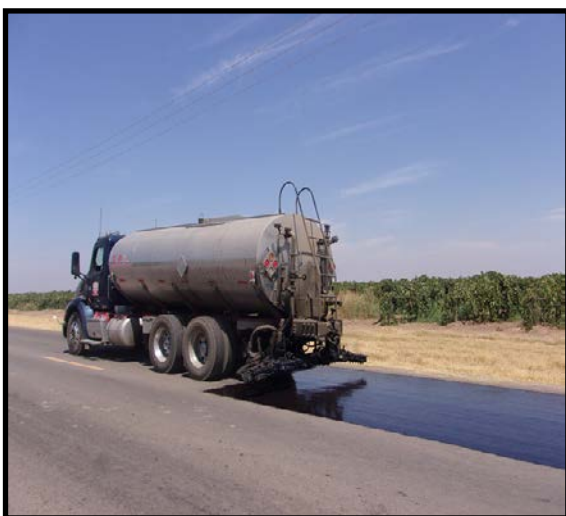
Spraying the oil on the roadway
