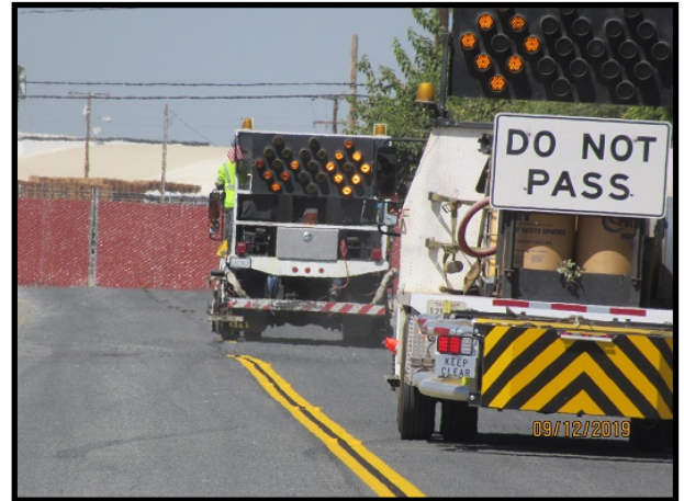
Centerline striping after chiprock sweeping
