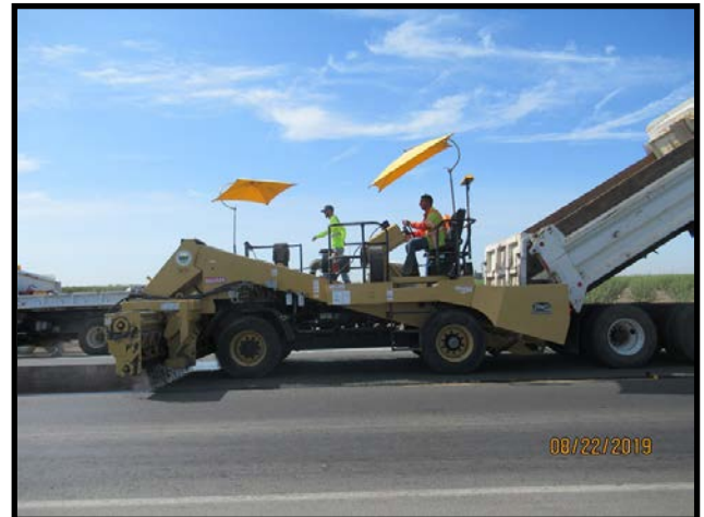
Chip Spreader placing rock over oil
