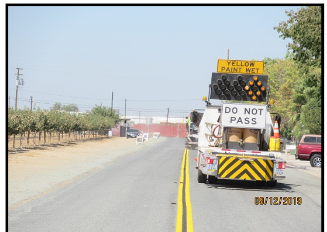
Striping/stencil crew repainting the centerline Stripe
