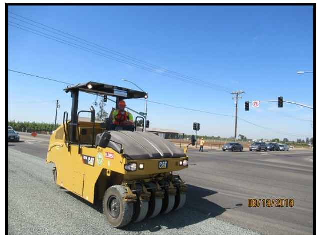
Rollers embedding the newly placed rock into the oil
