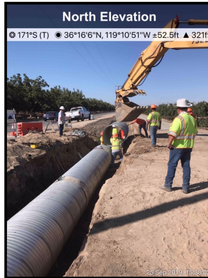
Installing new pipe
