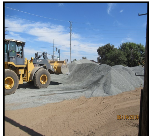
Begin loading the chipseal rock into trucks
