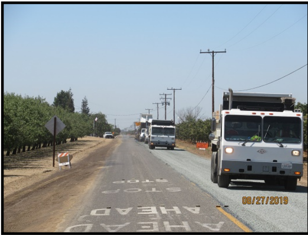
Transporting the rock to the Chip Spreader
